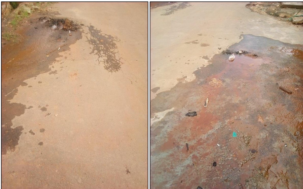
FIGURE 1: 1 DEFECTS OF UTILITY CUT ON THE PAVEMENT
