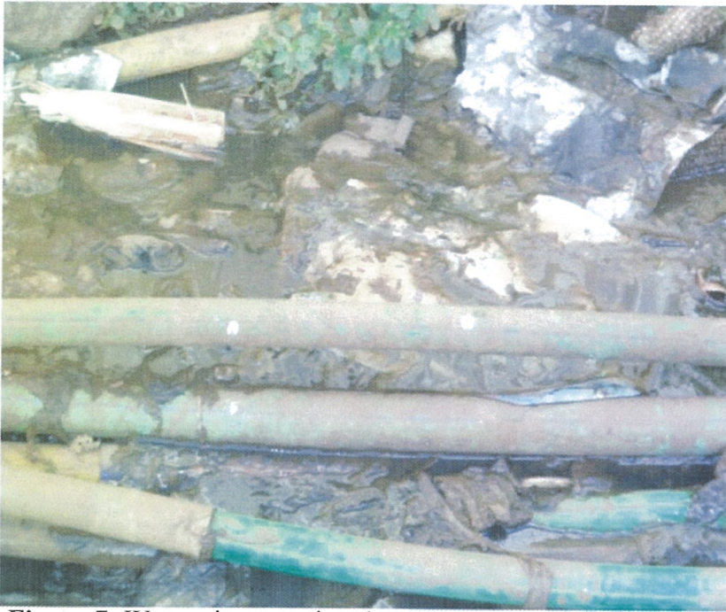
Figure 7: Water pipes passing through stagnant water in Mbuya
